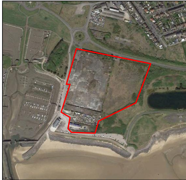
Photograph 1 (Extract from Google Earth – June 2021)
