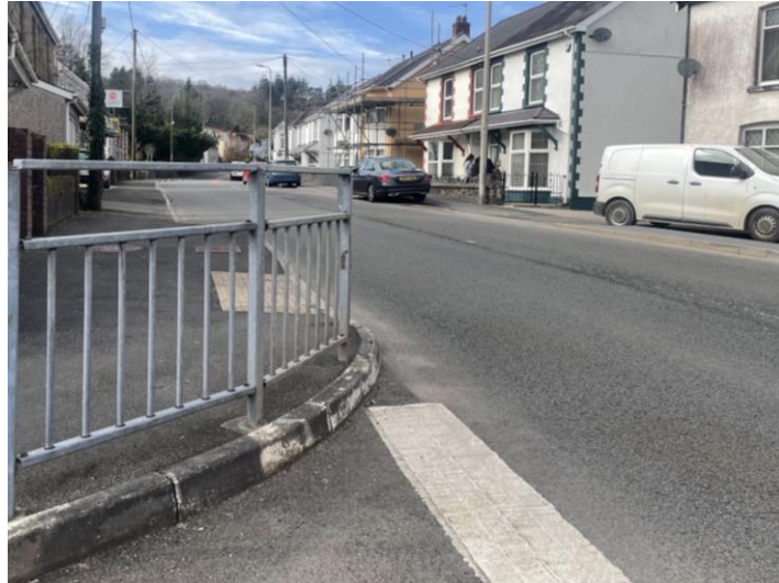
Photo 4 – view to left / north-west at junction with A483 road with wide visibility extending for well over 150 metres along Trunk Road from a 2.4 metres setback
