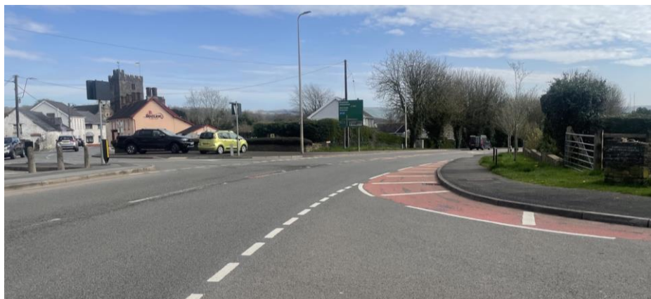
Photo 4 – view to right / south-east at junction with A483 road with wide visibility and separation distance to junction opposite into village centre
