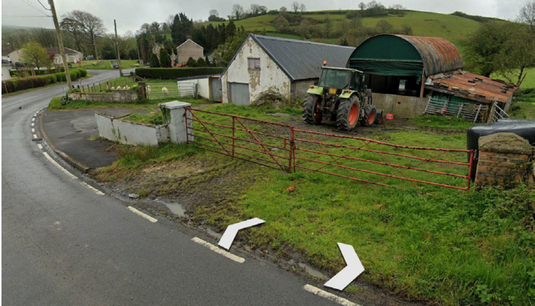
Figure 3 – Existing outbuildings as viewed from public highway upon Streetview (April 2022)
