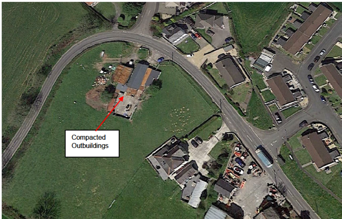
Figure 2 – Extract from Google Earth (April 2021) illustrating the existing outbuildings
