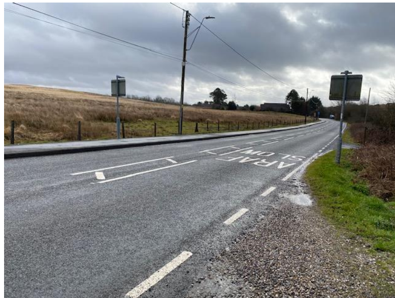
Photo 4 – view to right (east) from existing access onto A4068 road illustrating excellent visibility
