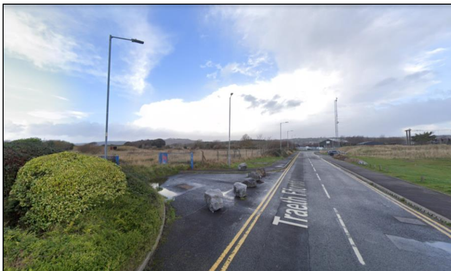
Photograph 2 (Streetscene of Traeth Ffordd)
