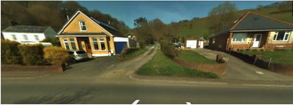
Photograph 2 – view from Gwscwm Road carriageway looking at existing access track
