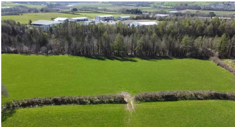
Photo 3 – aerial viewpoint looking west at A48 landscaped embankment, wholly screening views of the site from the A48 and Parc Pibwrlwyd
