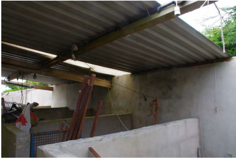
7. Interior of derelict building
