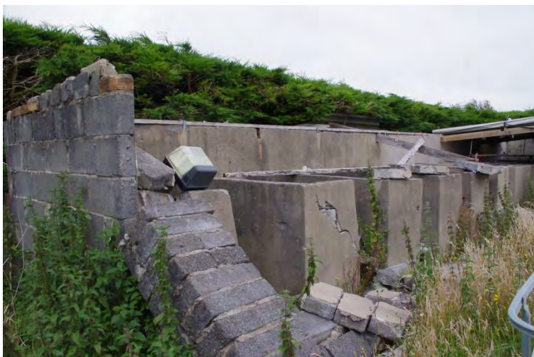
6. Northern end of building
