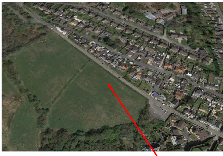
Fig. 7 – General aerial view of objection site
