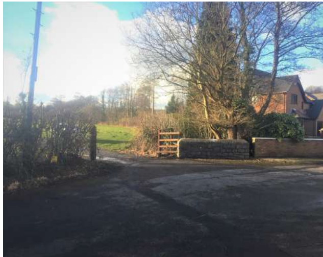
Fig 7: The existing site access on to Waunfarlais Road
